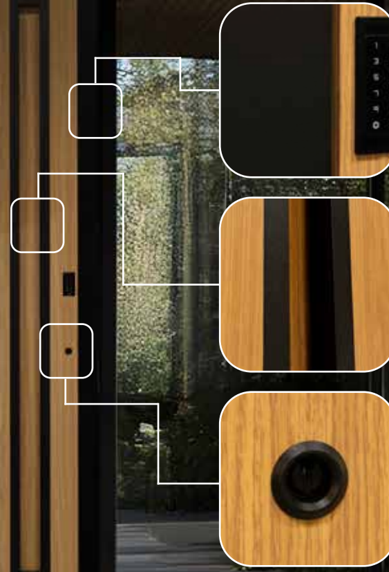
Black painted door frame
